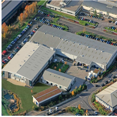
AESSEAL plc Group Headquarters, Rotherham, UK.
